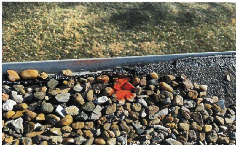
40. OVERVIEW OF SPLITS IN EDGE FLASHING
