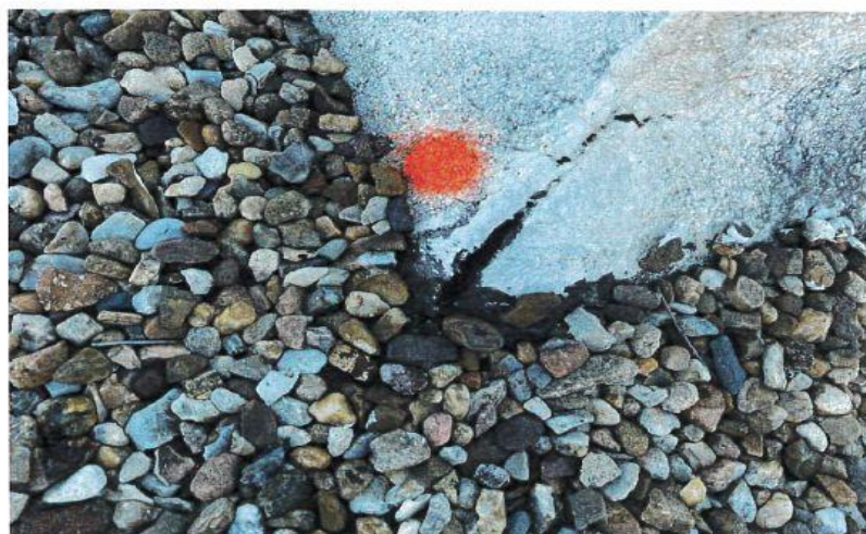
42. OPEN VOID IN CURB FLASHING SEAM
