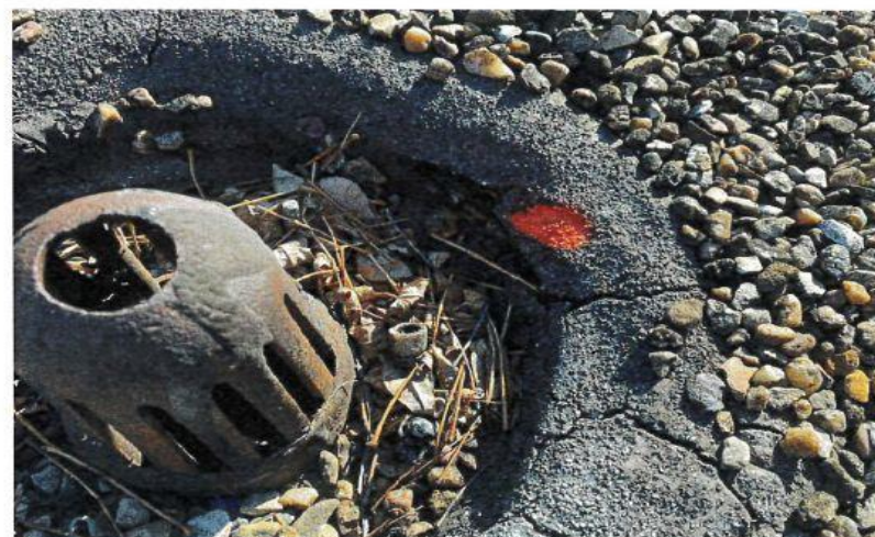
41. OPEN VOID IN DRAIN FLASHING
