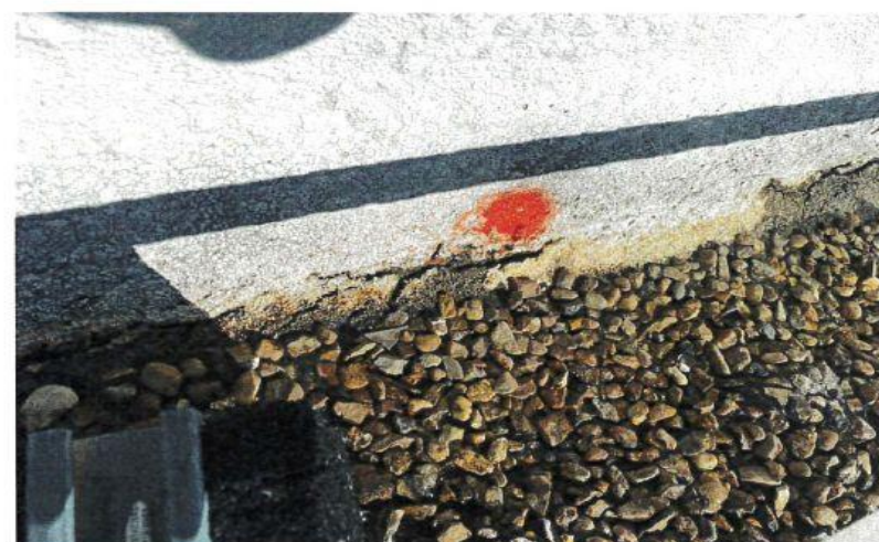
43. OVERVIEW OF DAMAGED CURB FLASHING
